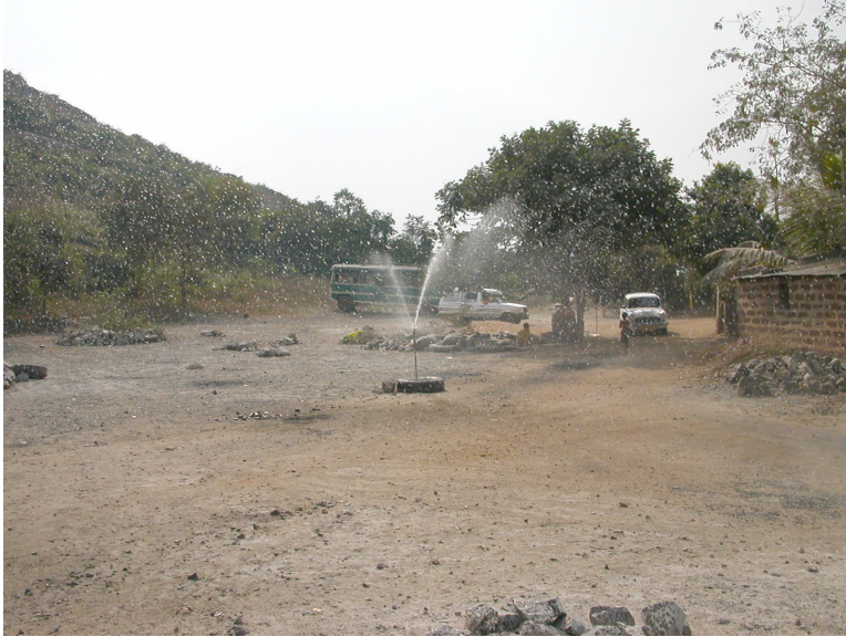
Figure 6. Sprinkler systems along roadways help to reduce dust created by trucks entering and leaving the facility.
