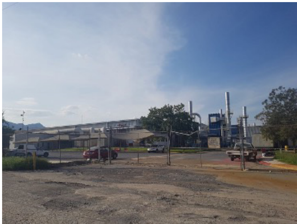
Figure 4: RIASA Grupo Gonher: South Fence Soil Lead Level of 1,600 ppm
