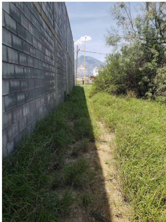
Figure 2: RECMAT de Mexico: East Wall Soil Lead Level of 1,800 ppm
